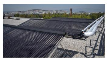
The "Zeosol" demo plant is a system for solar cooling and heating production which consists of a 12.5 kW adsorption chiller and a 30.0 kW backup compression
